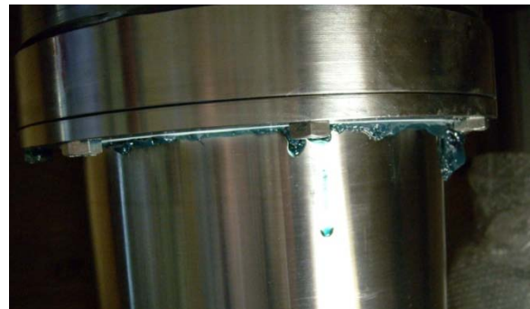
Shaft After Greasing
